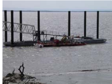
Placing the gang way in situ in preparation to be married up to barge (once commissioned)
