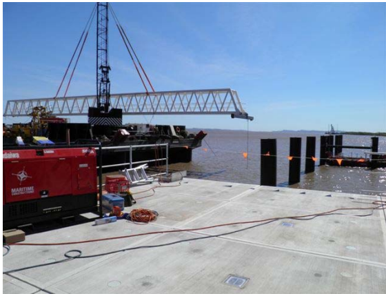
Placing the gang way in situ in preparation to be married up to barge (once commissioned)
