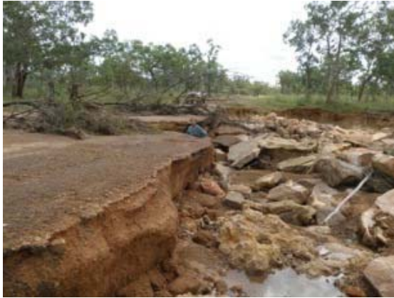
Between Gibb River Road and Drysdale River Station Damaged from March flooding event
