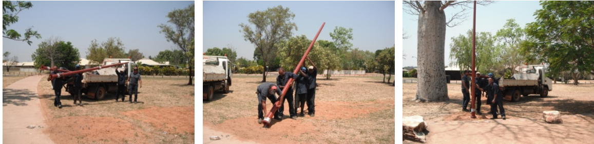
Installation of Nicolson Park Solar Safety Lighting
