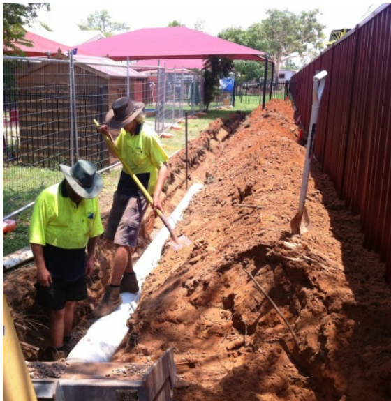
Installation of Drainage at Ewin Childcare Centre
