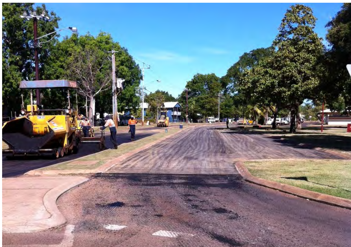
Asphaltting overlay on Konkerberry Drive, Kununurra
