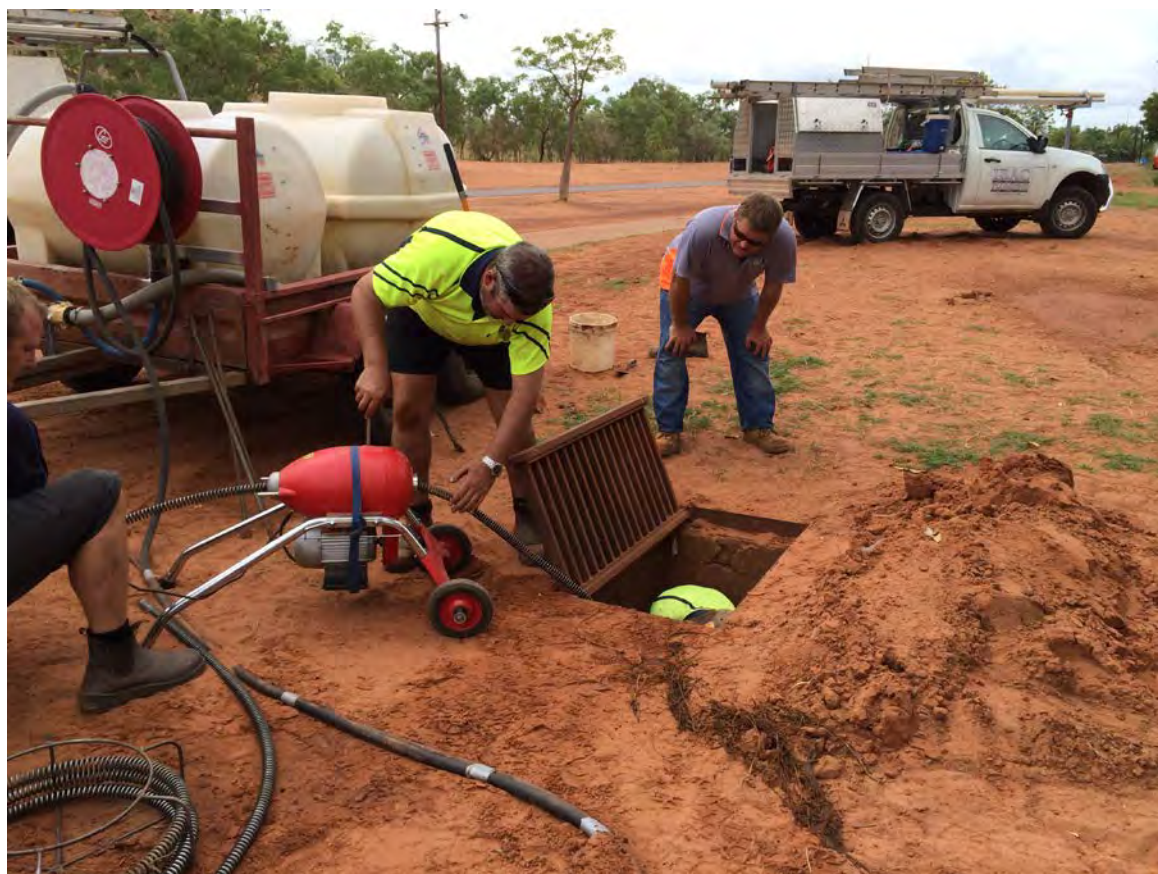
Cleaning of drains to assist with stormwater management
