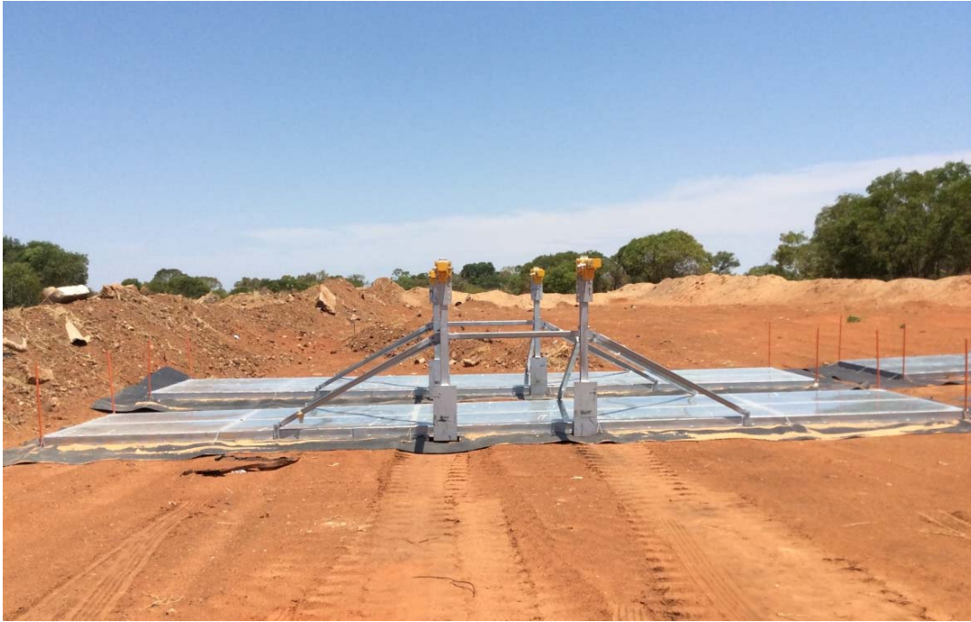
New temporary landfill covers in use at the Kununurra landfill site
