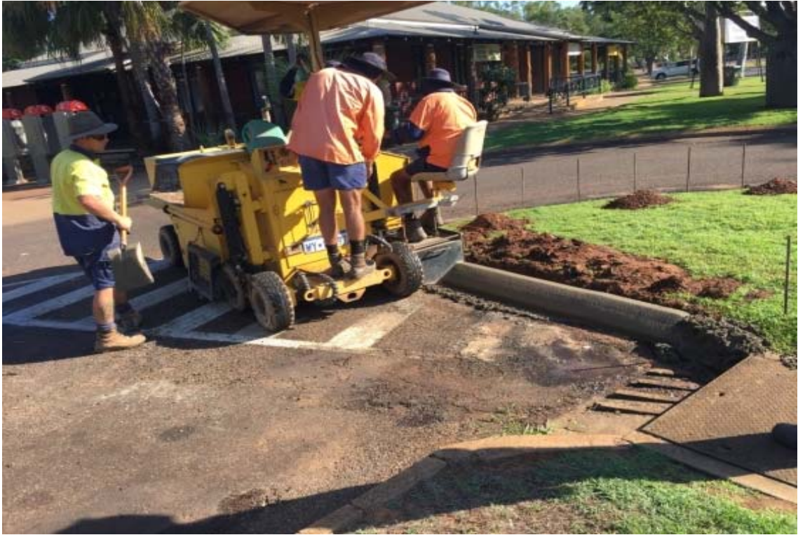
Replacement of damaged kerb – Kununurra
