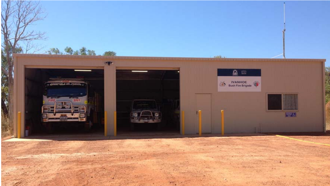
New Fire Shed
