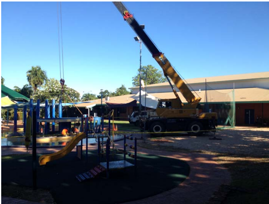
Removal of adventure pool platform
