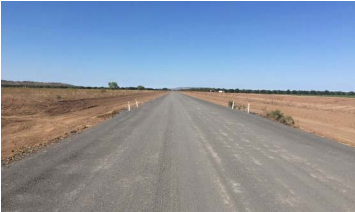
Re-sheeting – Carlton Hill Road
