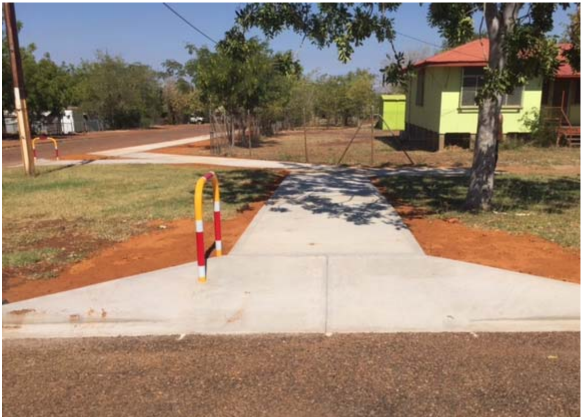
Installation of footpaths – Wyndham
