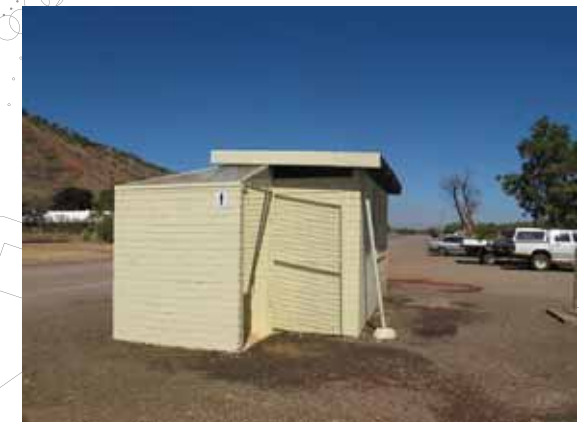
remove & relocate toilet facilities
