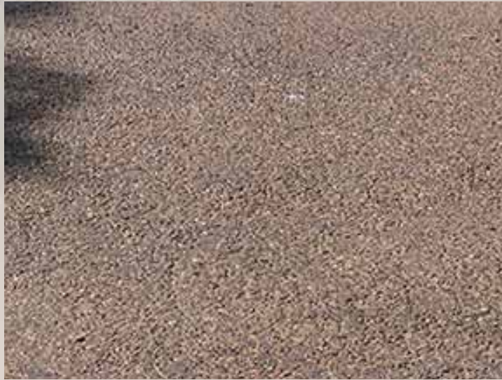
bitumen spray & aggregate
