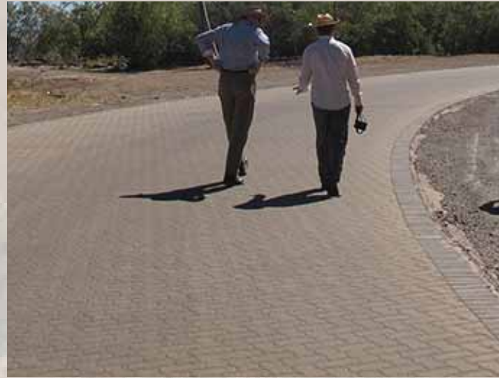
interlocking concrete brick paving - is subject to extreme inundation yet has performed well
