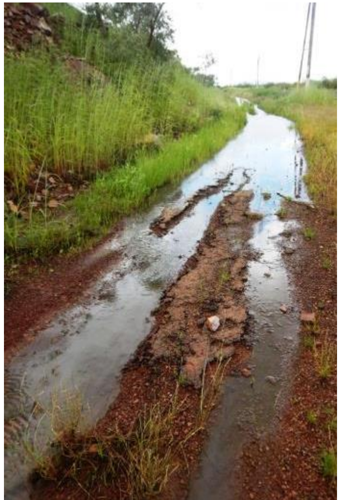
Image 19: Extensive Damage to Wyndham Port Path
